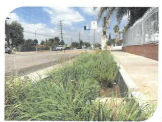
series of bioretention swales along Laurel Canyon Boulevard between Kagel Canyon Street and Terra Bella Street with curb, gutter, and sidewalk improvements. This project collected stormwater runoff from a 125-acre drainage area. CWE provided preduring, and post-construction support for this project.
