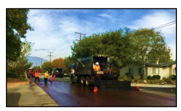
Temple City Citywide Pavement Rehabilitation **Project (\$900K):** This project included citywide construction of slurry seal to various streets. Transtech provided management of City's pavement management system, project design, construction management, and inspection services.
