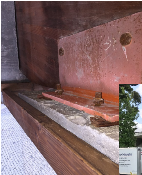
Figure 6: LOOSE BOLTED CONNECTION
