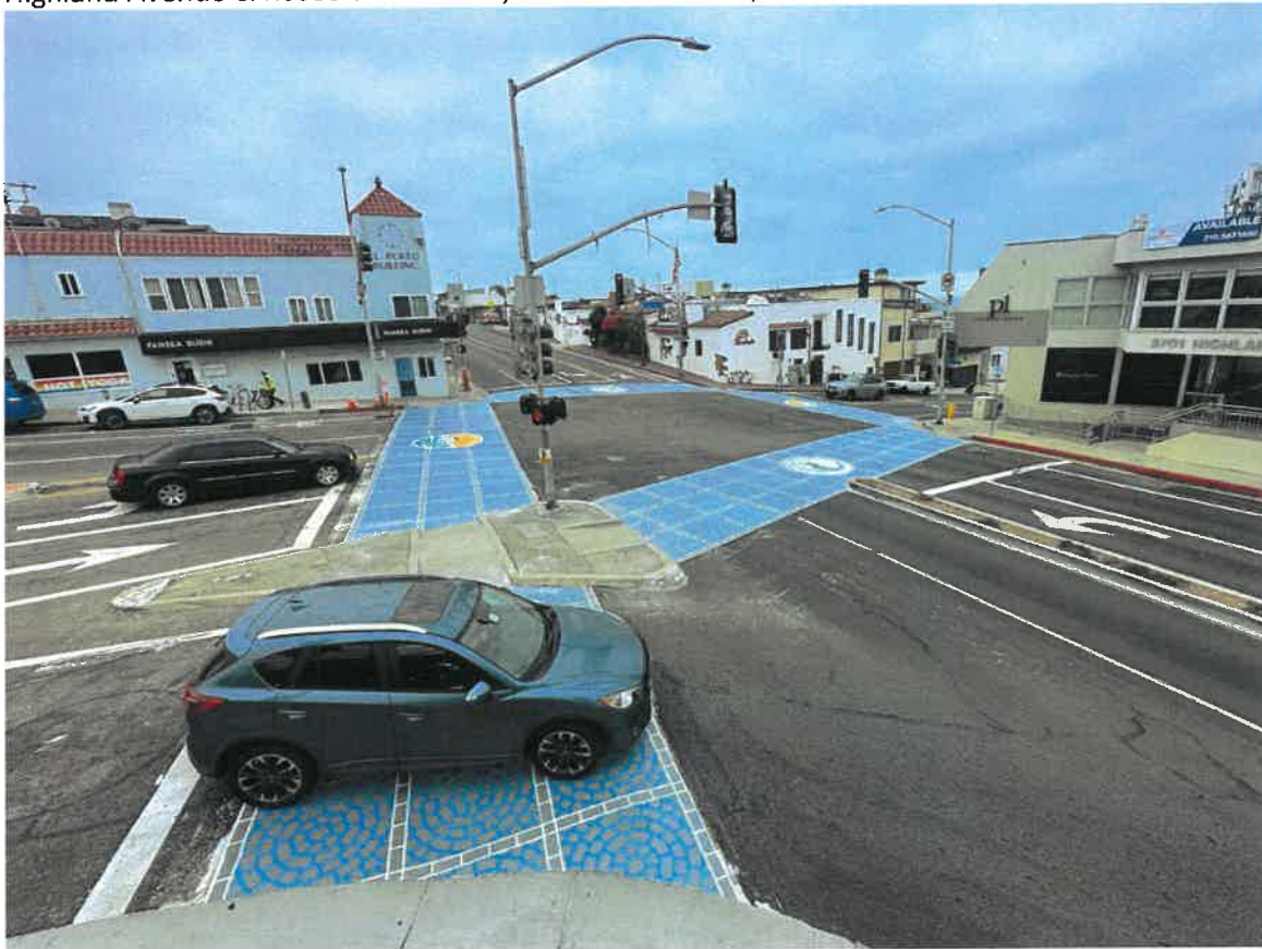
City Logo Crosswalks - Thermoplastic Installation by Shariden Design Asphalt Highland Avenue & Rosecrans Avenue, Manhattan Beach, CA - June 2023
