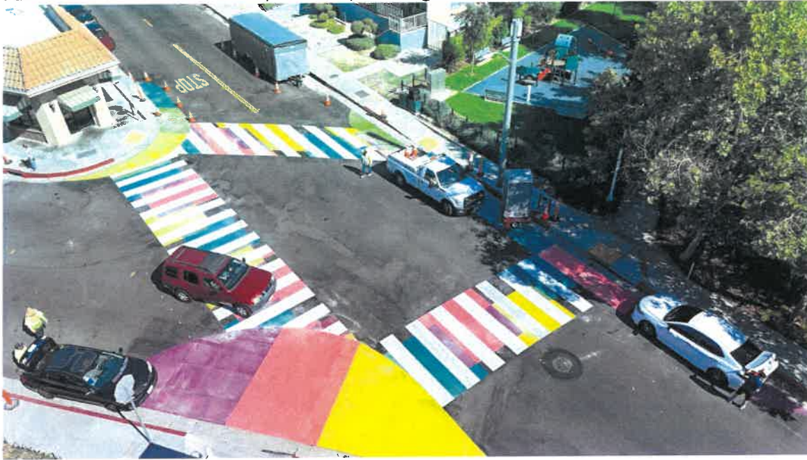
City Logo Crosswalks - Thermoplastic Installation by Shariden Design Asphalt Highland Avenue & Rosecrans Avenue, Manhattan Beach, CA - June 2023
