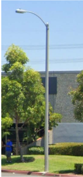
CONCRETE POLE (SCE)
